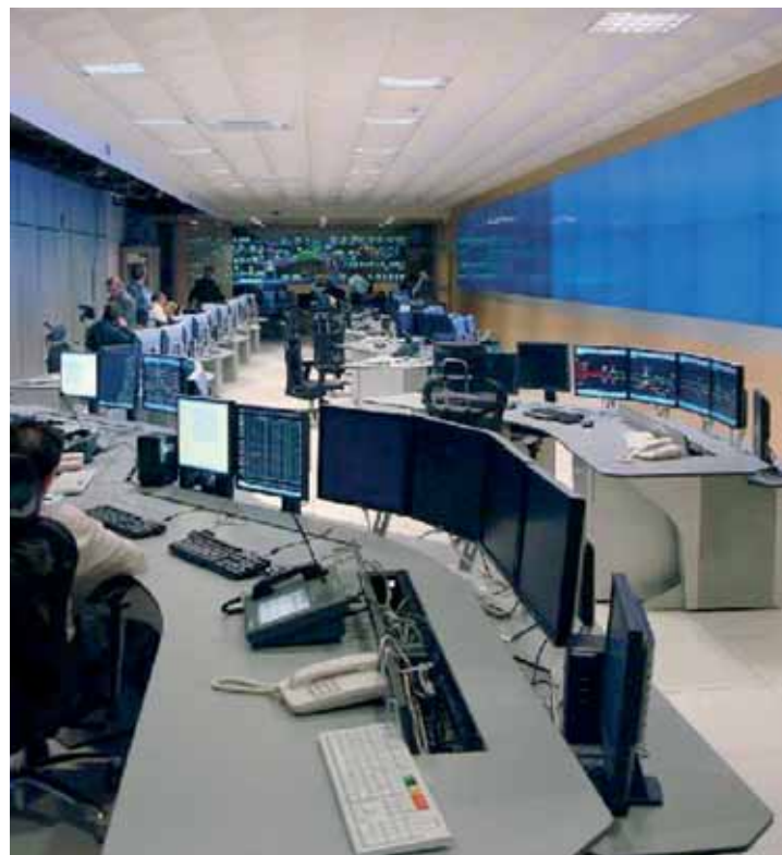
Traffic Control Centre
